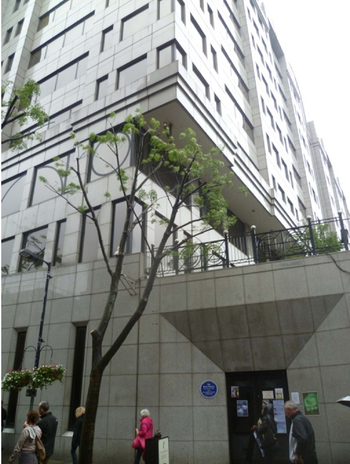
Figure 2.9 Picture of the Rose Theatre building as it stands now (Picture taken in June 2012). The door on the bottom right hand leads to the basement where the theatre remains are preserved.
